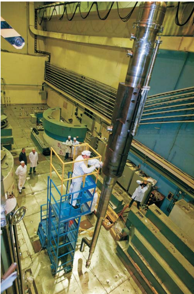
Frank Laboratory of Neutron Physics. In the frames of the IBR-2 refurbishment programme, a new reactor shell has been received from the Dollezhal Research and Development Institute of Power Engineering and installed in the reactor hall
