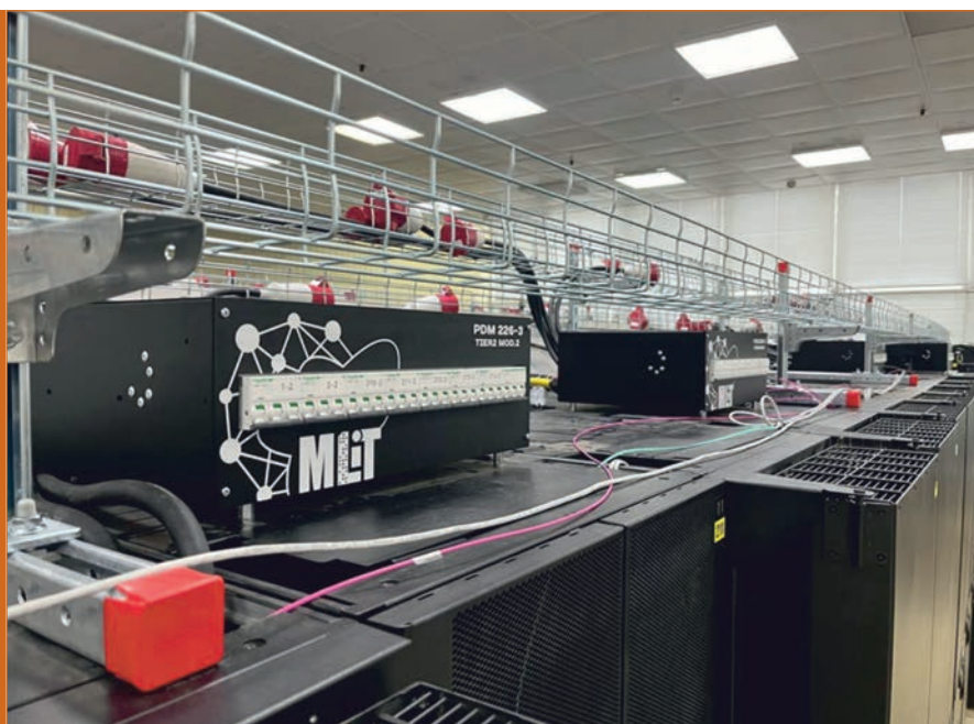
Power distribution modules (PDMs) developed at MLIT and installed at the MICC
