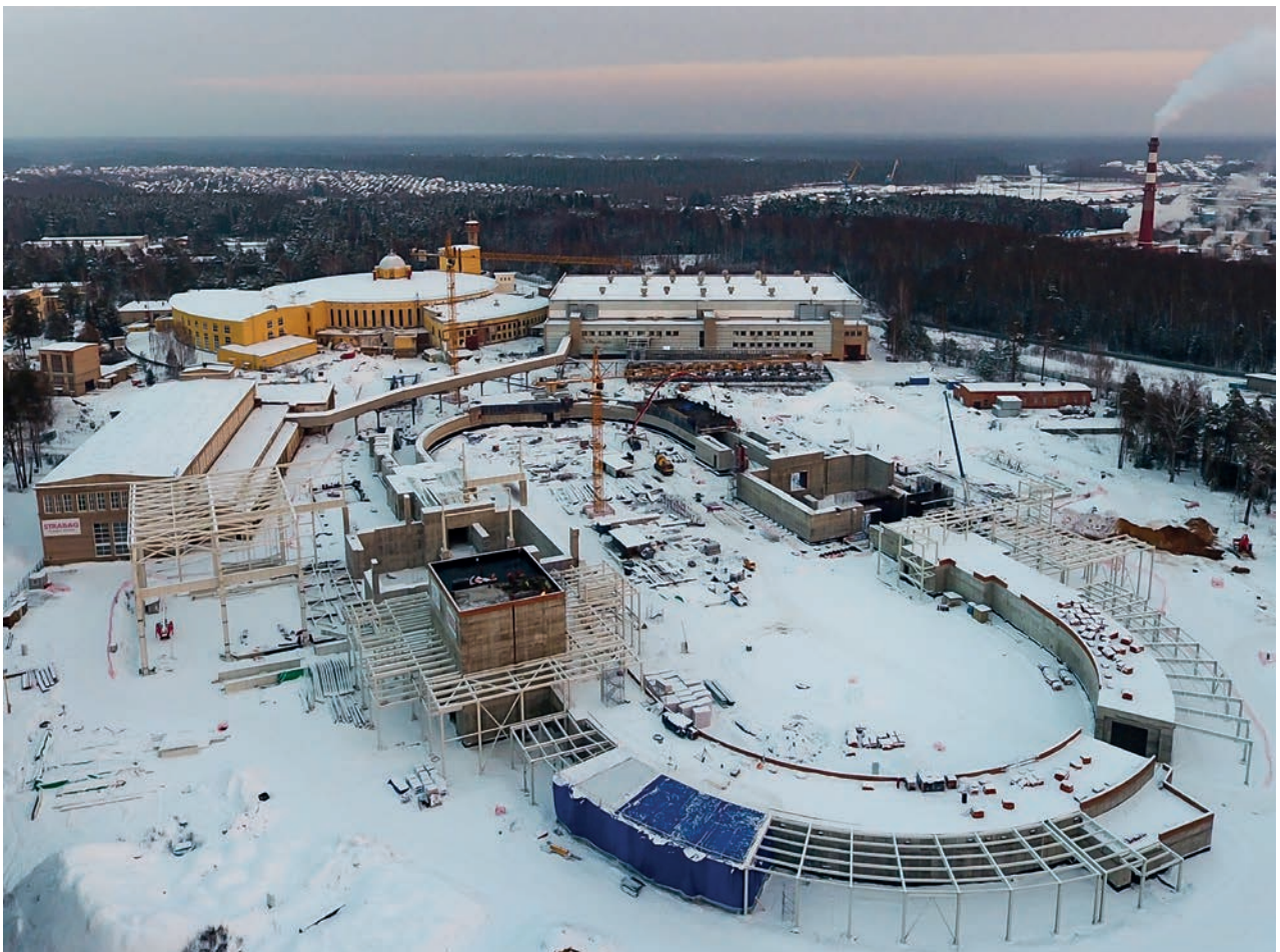
The construction site of the NICA complex
