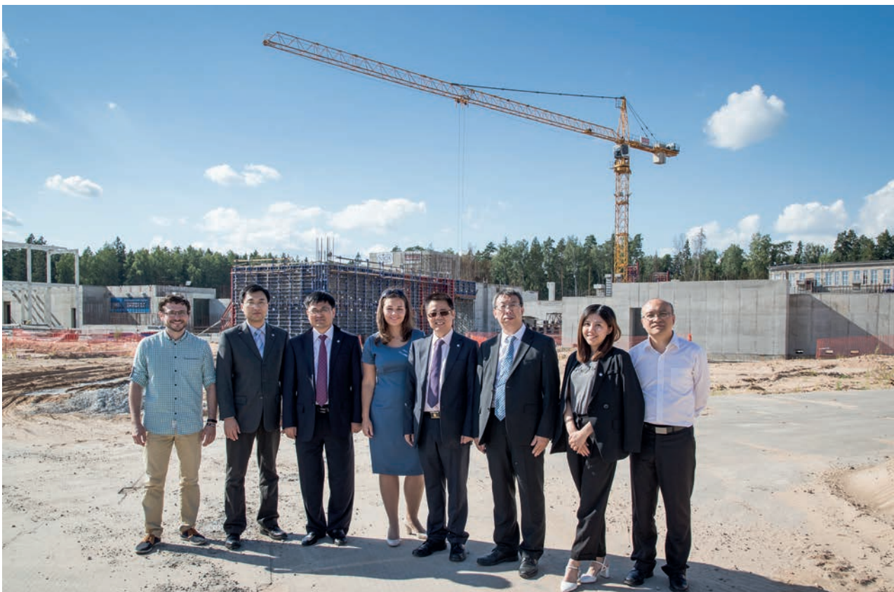
Dubna, 10 August. The delegation of the China National Nuclear Corporation and the China Institute of Atomic Energy visits the NICA construction site
